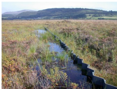
Plastic piling raising water levels in an old peat cutting, Cors Fochno, Ceredigion. Photo: P. S. Jones.
