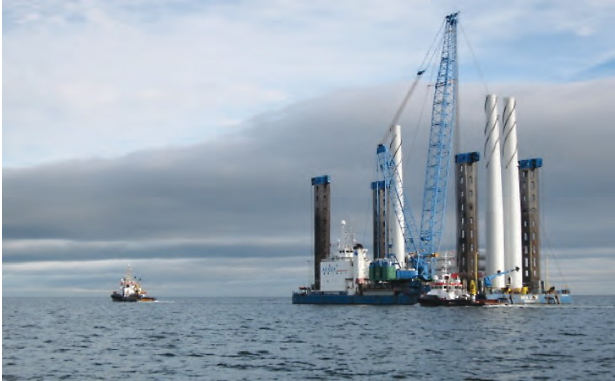
Figure 4 Windfarm jack up rig outward bound under tow from the port of Mostyn through the Mostyn Operational Area.
