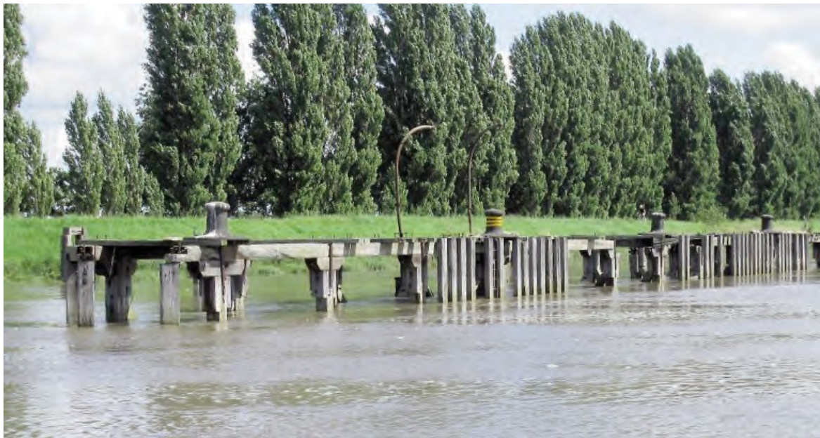
Figure 12 Disused jetty on the north bank of the river upstream on Hawarden Rail Bridge
