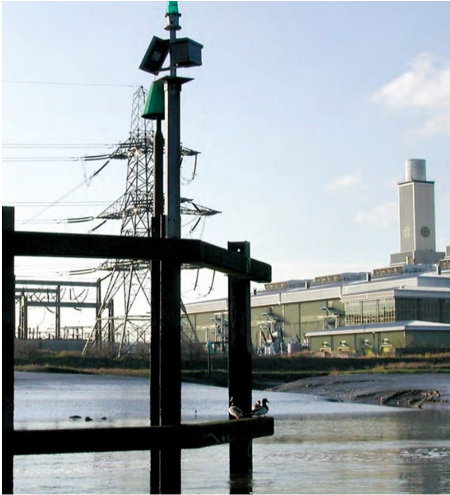
Figure 7 South training wall light structure.
