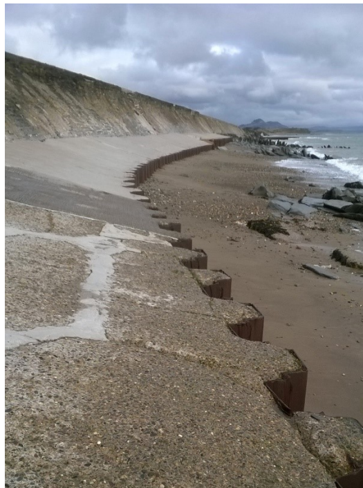
Figure 10 Coastal defences, North Wales. Photo: Heather Lewis
