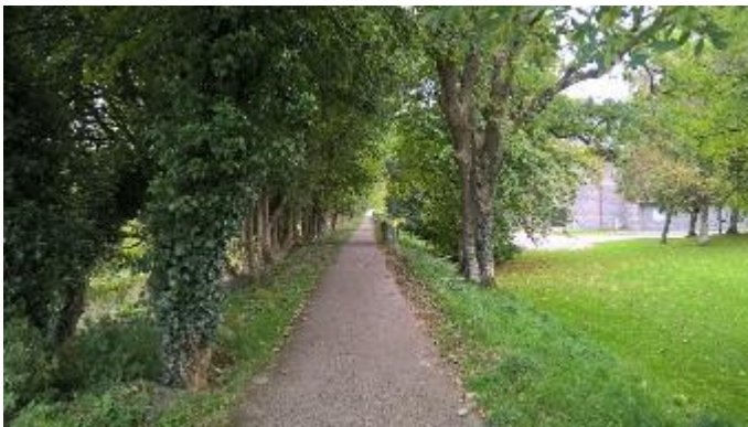
PICTURE 25. TREE TOPPED EMBANKMENT
