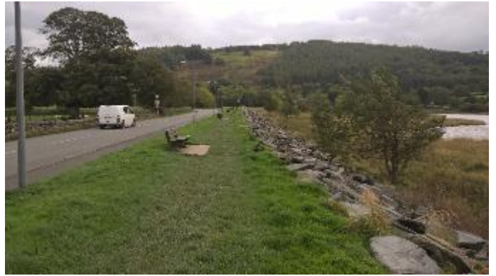
PICTURE 14. STONE FACED FLOOD BANK. TN16.
