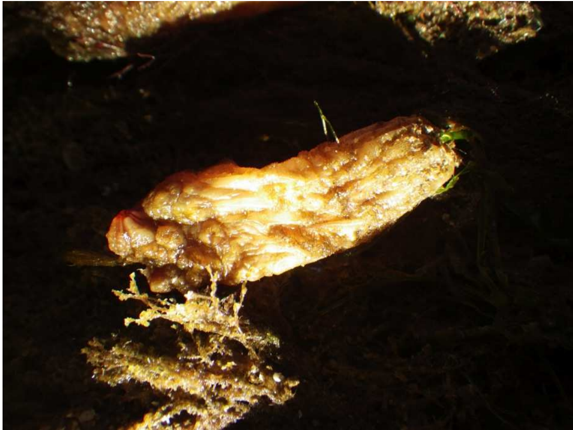
Figure 7. The invasive Styela clava on concrete slipway at Abersoch lifeboat station.
