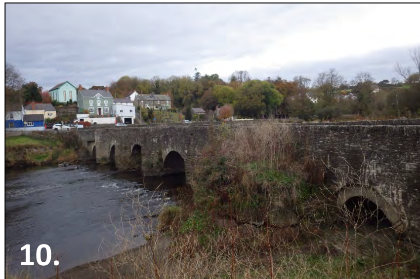
Image 10: An example of a major in-channel structure (Site ID 25334)
