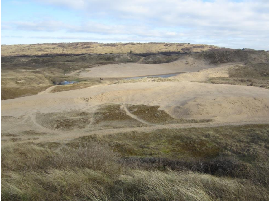
Photograph 13. View north-eastwards across the Phase II works
