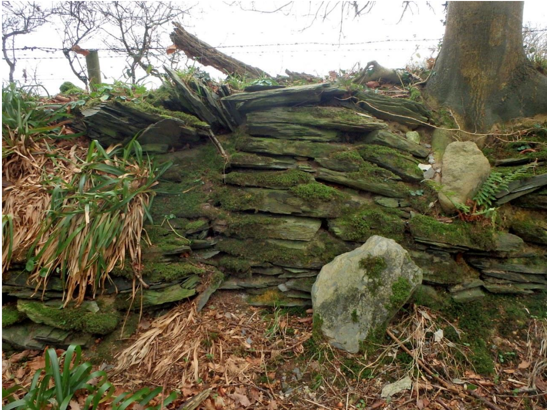
Fig. 26. Old field wall at top of Compartment 4, probably built from stone quarried nearby in the woodland.
