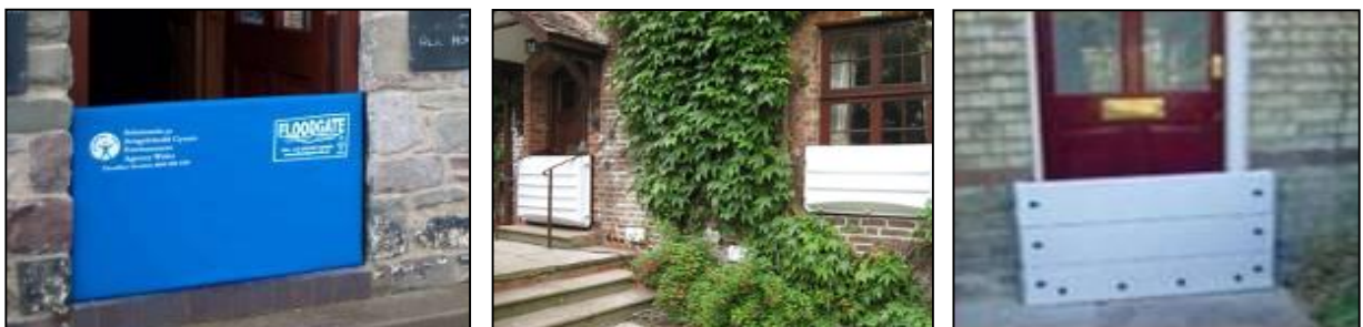
Figure 9 Examples of Individual Property Protection measures
