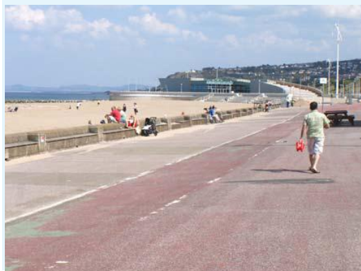
Figure 7 coastal defence and regeneration works at Colwyn Bay, Photo/Image courtesy of BCA Landscape
