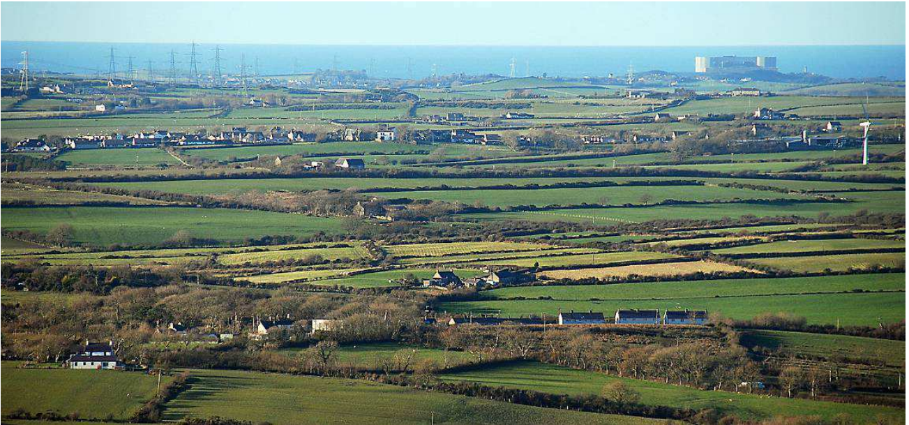
North Anglesey – the pattern of Medieval or earlier farm buildings and field boundaries in this predominantly open and still rural landscape are punctuated by more recent features: modern housing, pylons, wind farms, and the nearby Wylfa Power Station. © John Briggs
