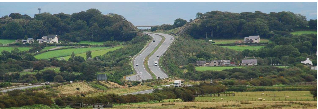
The A55 road crosses the area, here seen running over the low hill ridge SE of Malltraeth marsh, near Gaerwen. © John Briggs
