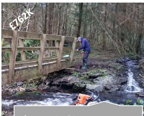
a) Practical improvements on the ground
