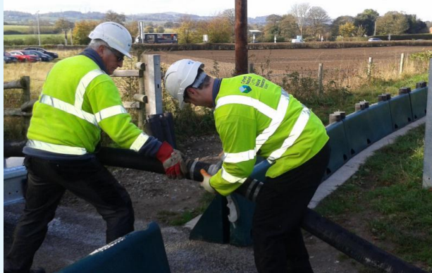
Fig 13: NRW officers erecting demountable defences.
