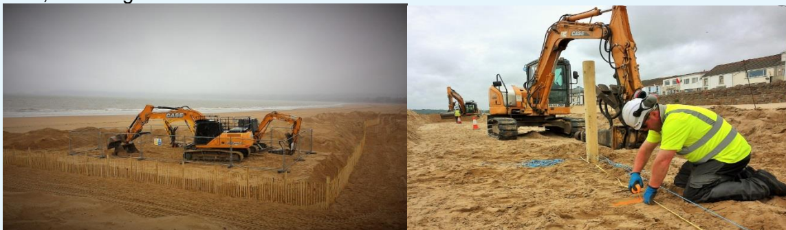
Fig 12: dune stabilisation works, Swansea
