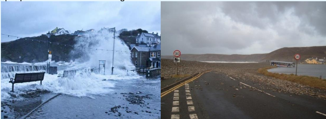
Fig 8: Flooding at Newgale (Credit: Pembrokeshire County Council)
