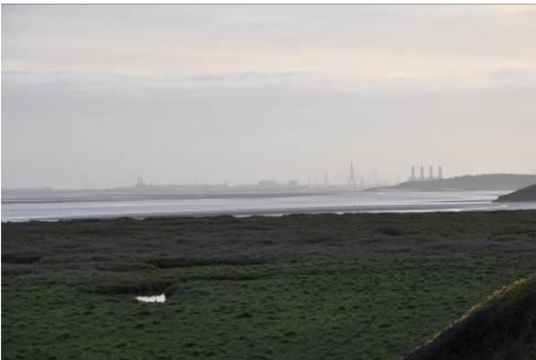
Deeside Power Station
