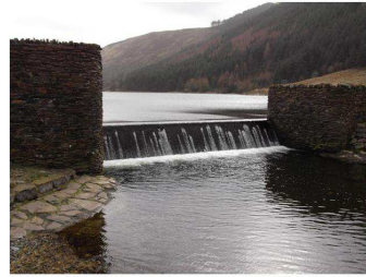
Weirs and in-channel structures
