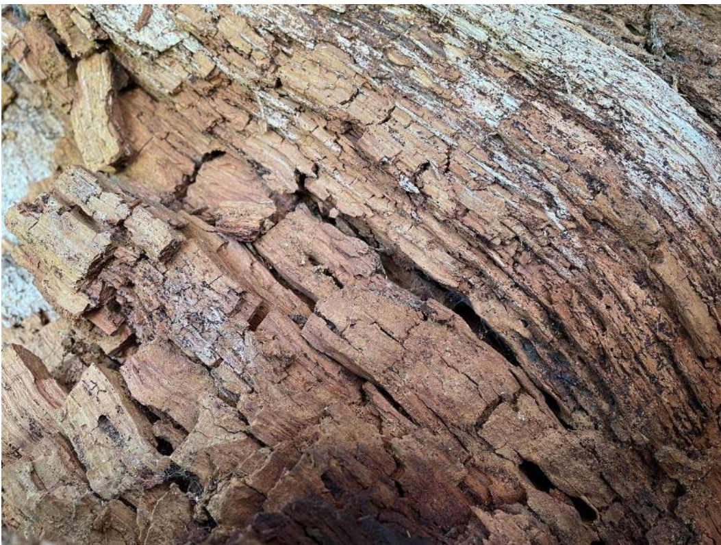
Photo A1.9. Flight interception trap location 5. Red-rotten wood on the trunk of the oak at ST5273.9528 where a 4-bottle trap was operated, although the cavity entrance was too small to allow the trap to be placed inside.
